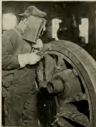
FIG. 5.—HEAVY REPAIRS ON LOCOMOTIVE DRIVING WHEEL BY ARC WELDER.
